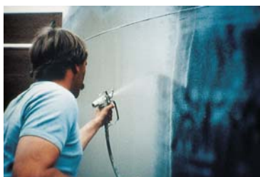
Posa in opera con airless.
